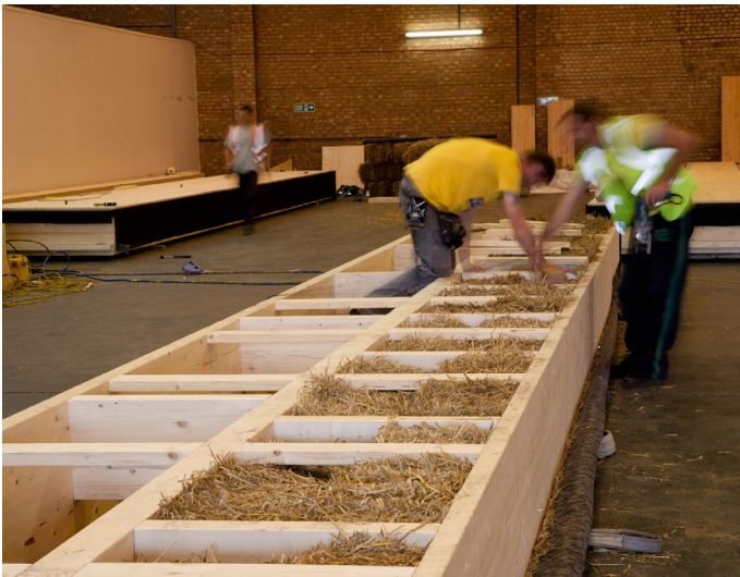
Fig 17: It takes straw bale construction one step further using straw within an external curtain wall system. (Make Architects, 2011)
